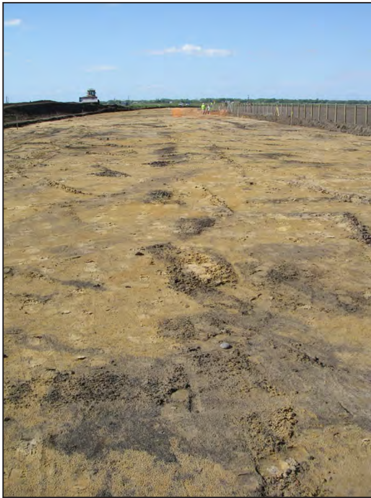
Plate 1. General site shot of stripped road corridor, looking northwest
